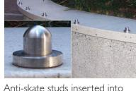
Anti-skate studs inserted into ground along spines of octagonal form, to mitigate anti-social behaviour.
